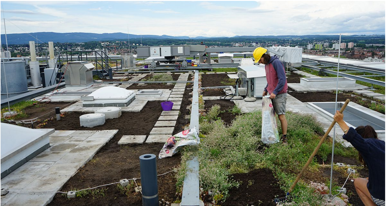
Figure 3: Greening the roof of the university building
