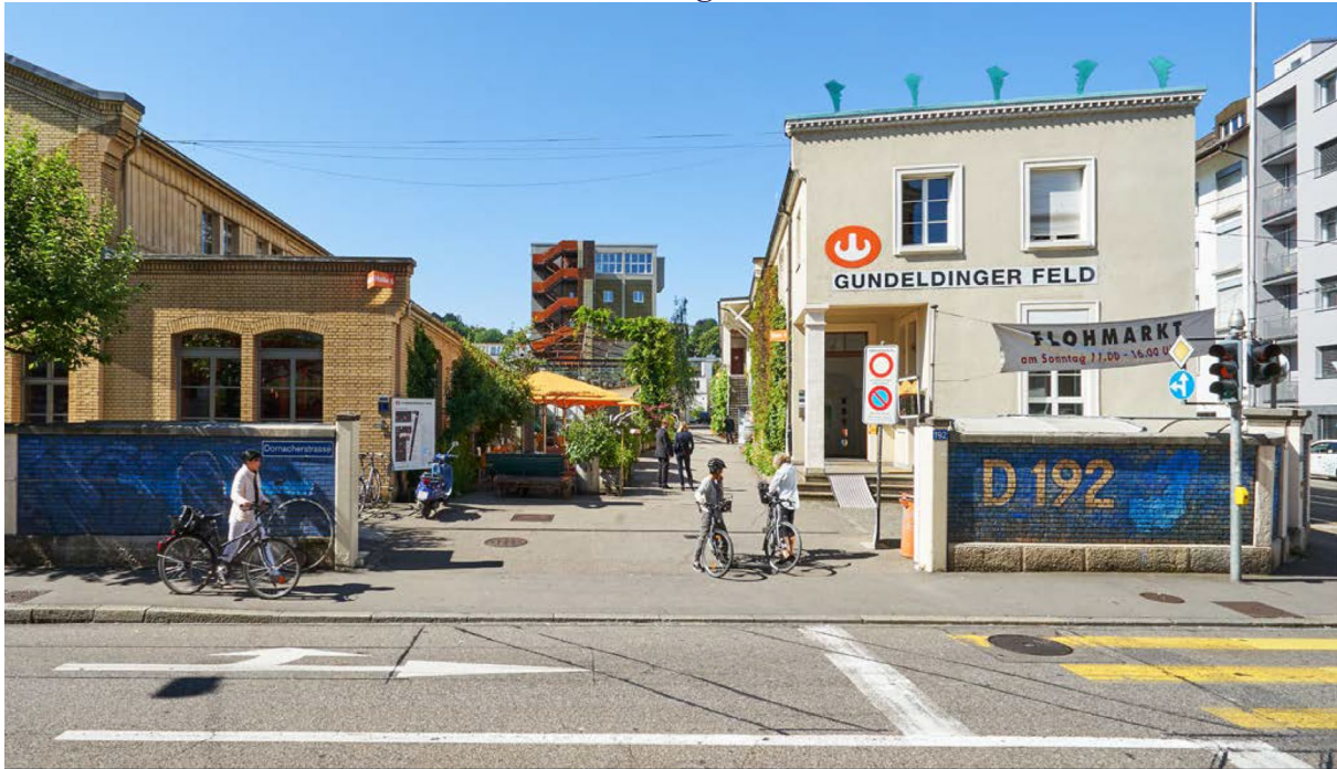
Figure 1: The northern entrance to the Gundeldinger Feld
