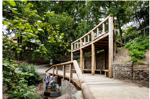
Figure 6: Renewed part of the park
