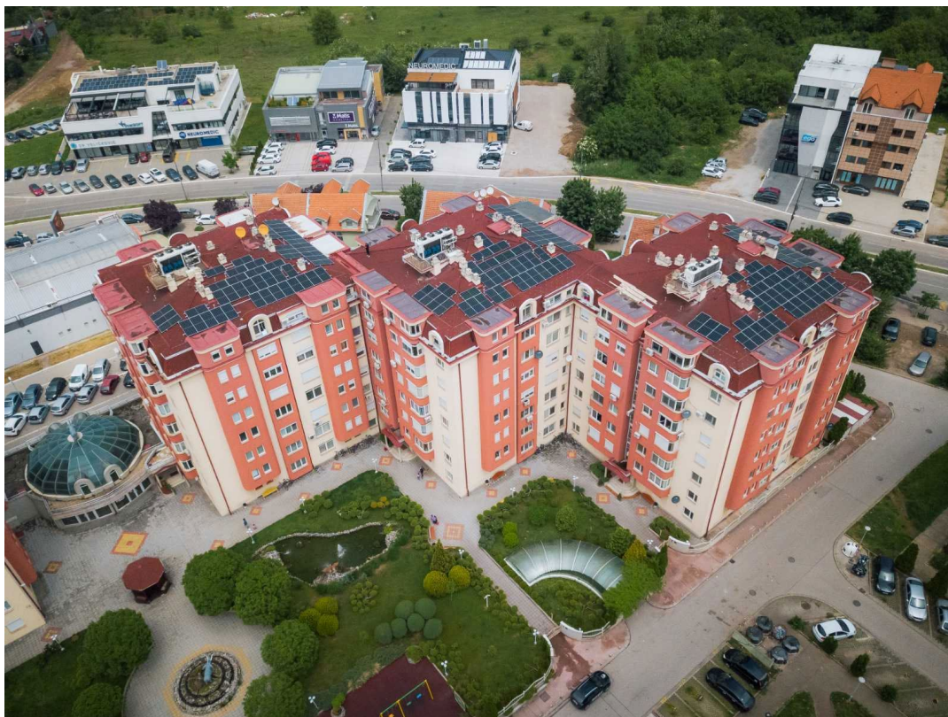
Figure 1. Magdon photovoltaic power plant. (Photo by Vladimir Rajski)
