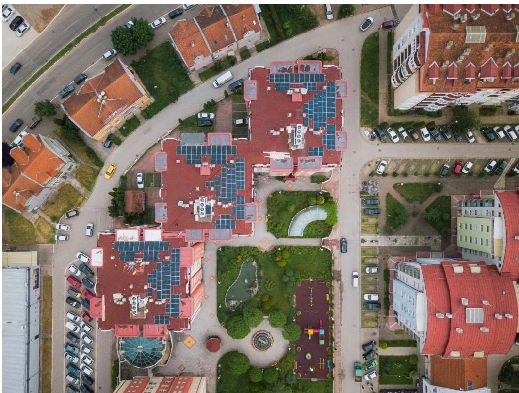
Figure 2. Magdon photovoltaic power plant. (Photo by Vladimir Rajski)
